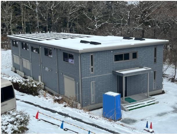
Completed high school dormitory/classroom
